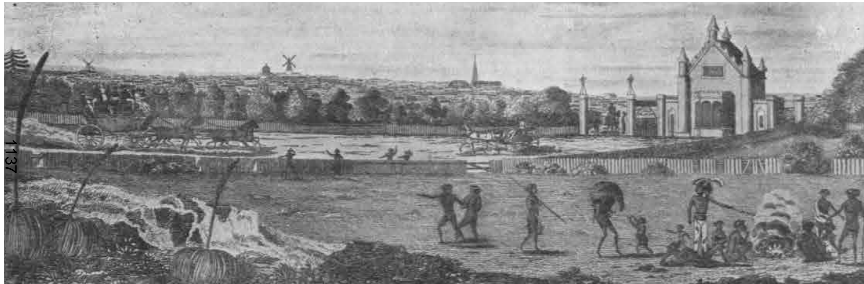
The George Street Toll Bar in 1829, looking northwards. From 1830 to 1900 subdivision and occupation of this area changed it to an urban form.
