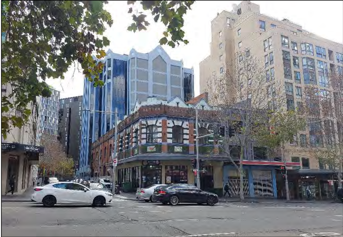
Figure 6 Site Viewed Looking North West from George Street Source: Mecone
