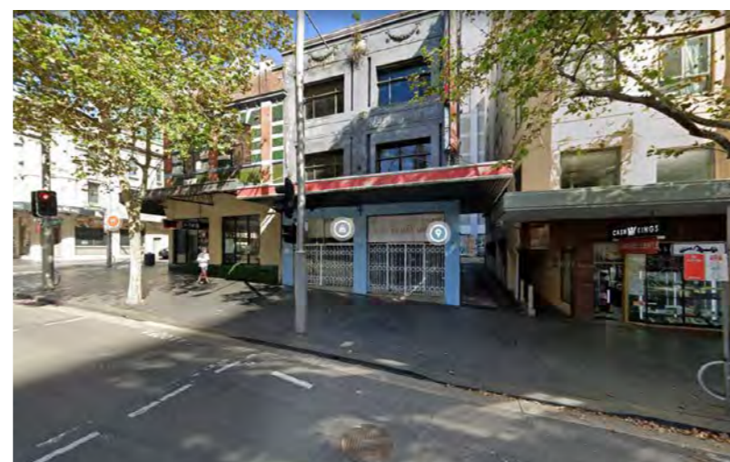
Pedestrian footpath from George Street with existing lane
