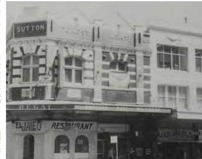
1979 - facade remains substantially in tact despite 1985 fire
