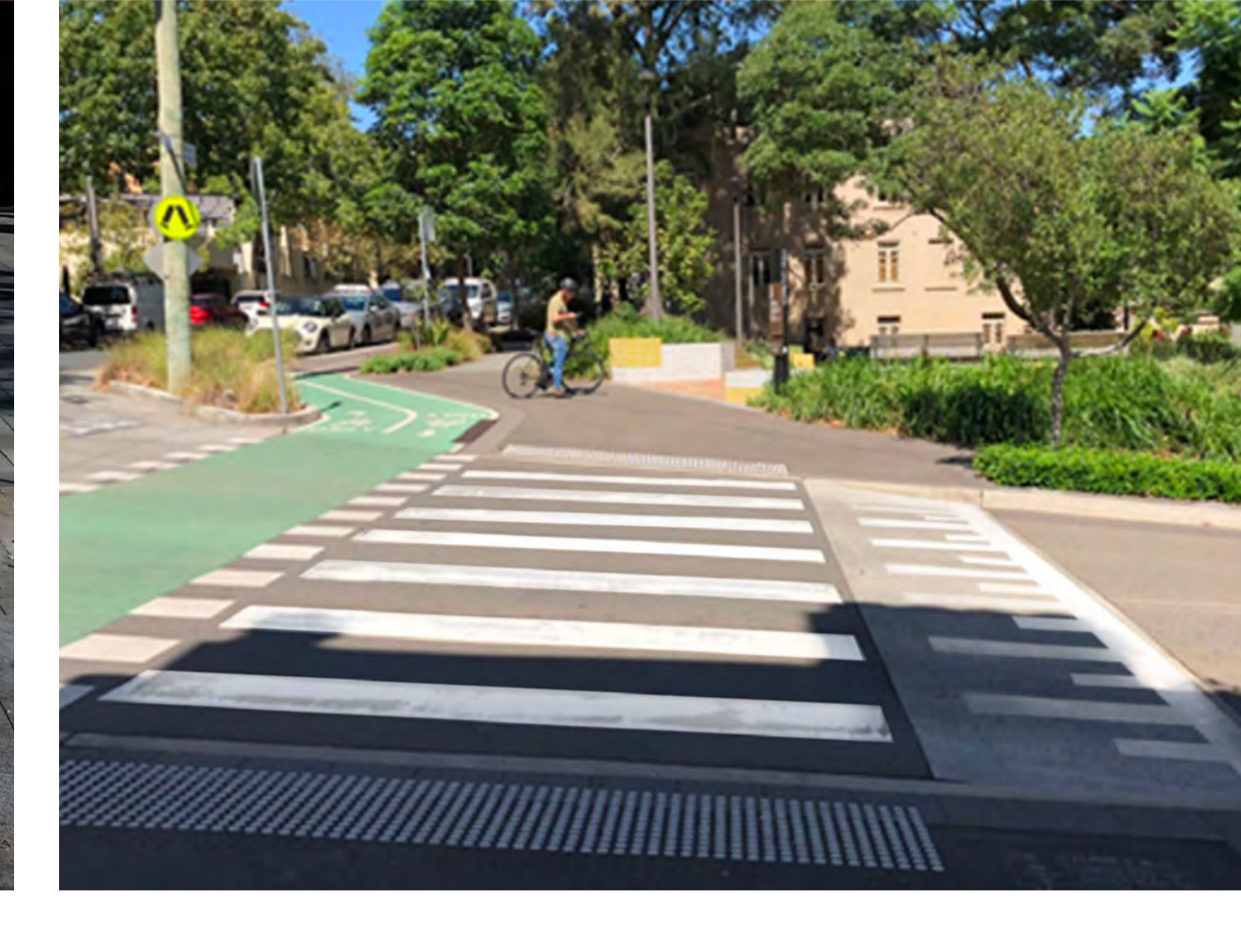
pedestrian crossing with adjacent bike crossing
