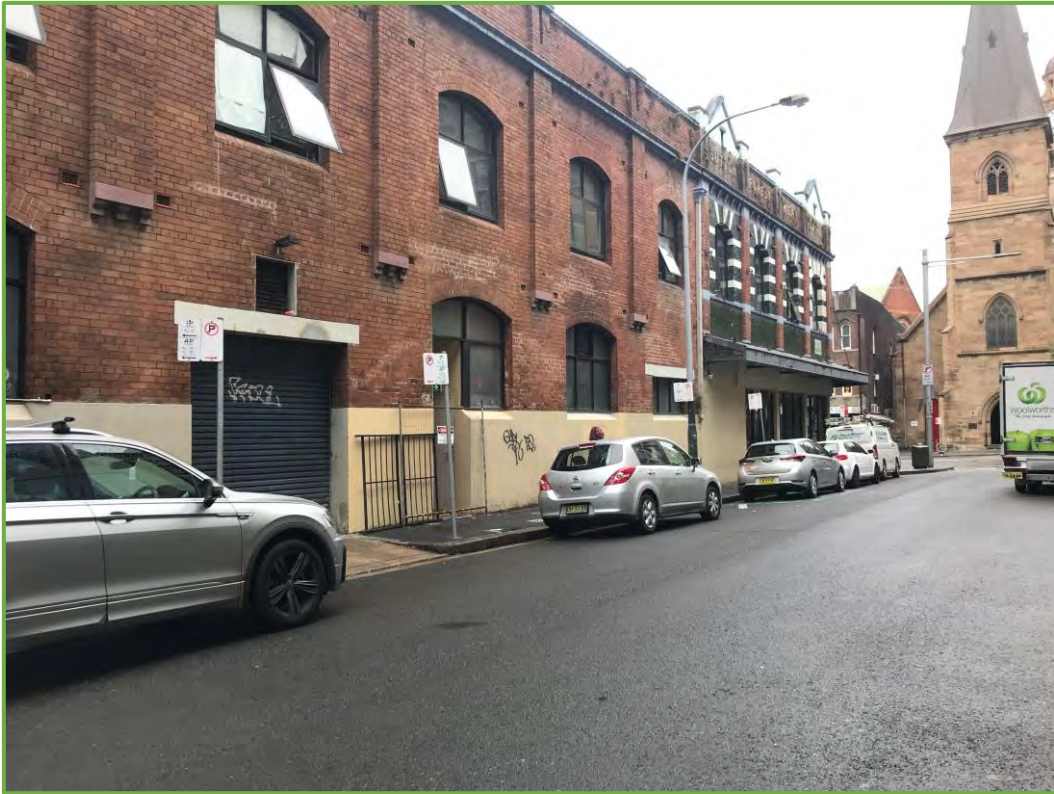
View looking east along Valentine Street at the site.
